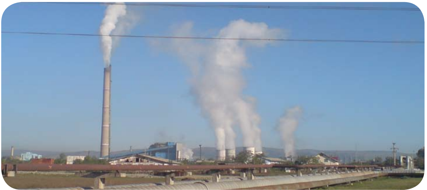
New improvement makes the district heating system in Drobeta Turnu-Severin more efficient.
